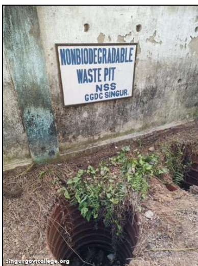
Separate pits for waste disposal at GGDC Singur
